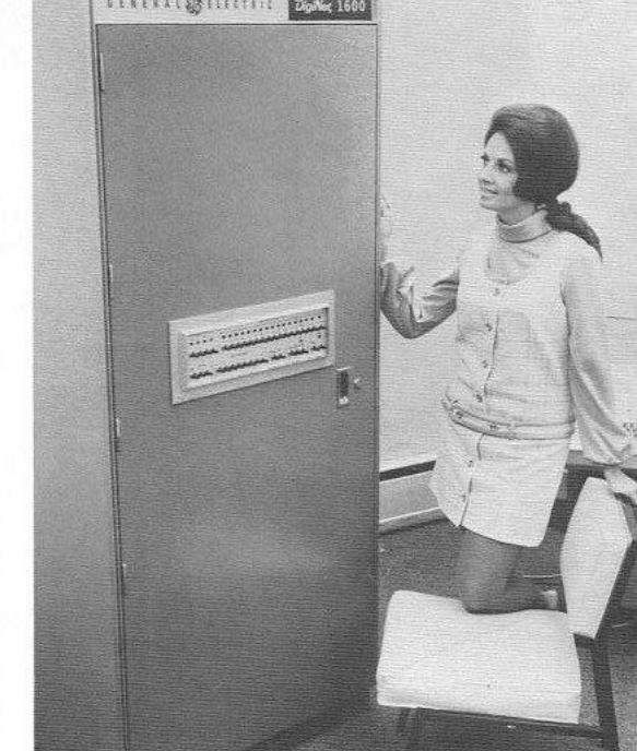
DigiNet 1600 data communications concentrator (produced by the Data Networks Operation of DCPD) aids time sharing companies and other remote-line computer users in trimming transmission costs. It's an answer to an industry need to make possible effective and economical combinations of computer power and communications power.
