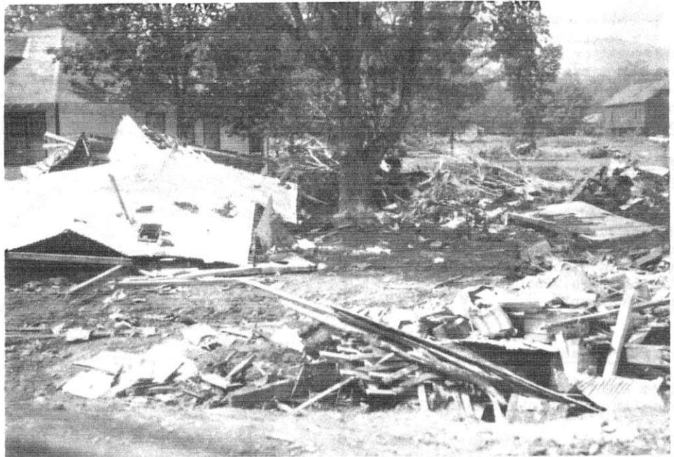
RUBBLE AT THE BRIDGE AT MASSIE'S MILL provides mute testimony of the destruction wrought by the flood waters in the early morning hours of August 20. Countless similar scenes exist.
