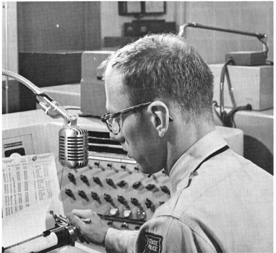
Shure Unidyne II unidirectional Microphone in typical base station use. (Note APCO Signal Card)
